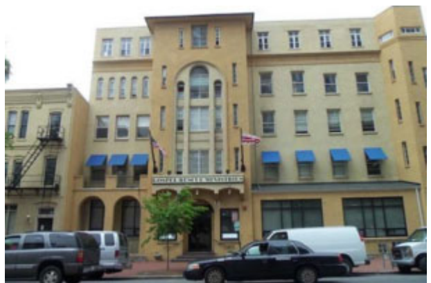
Rock Creek Property Group LLC has sold the former Gospel Rescue Ministries building for $28.5 million.
